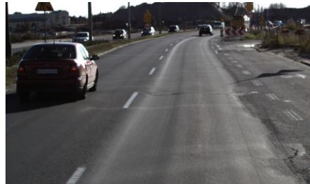
Figure 1: Pavement rutting observed on provincial road W719 in Warsaw, Poland
