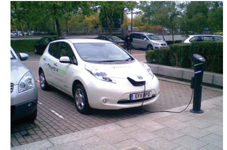
Figure 2: EV charging point in use at Milton Keynes city centre
